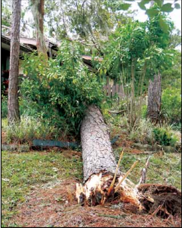
A tree rests on the roof of an apartment at Hillside Trace, 37975 Hillside Lane, after it was felled by Hurricane Irma.
